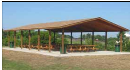
The new shelter at Fort Liberty Playland, constructed last summer.
