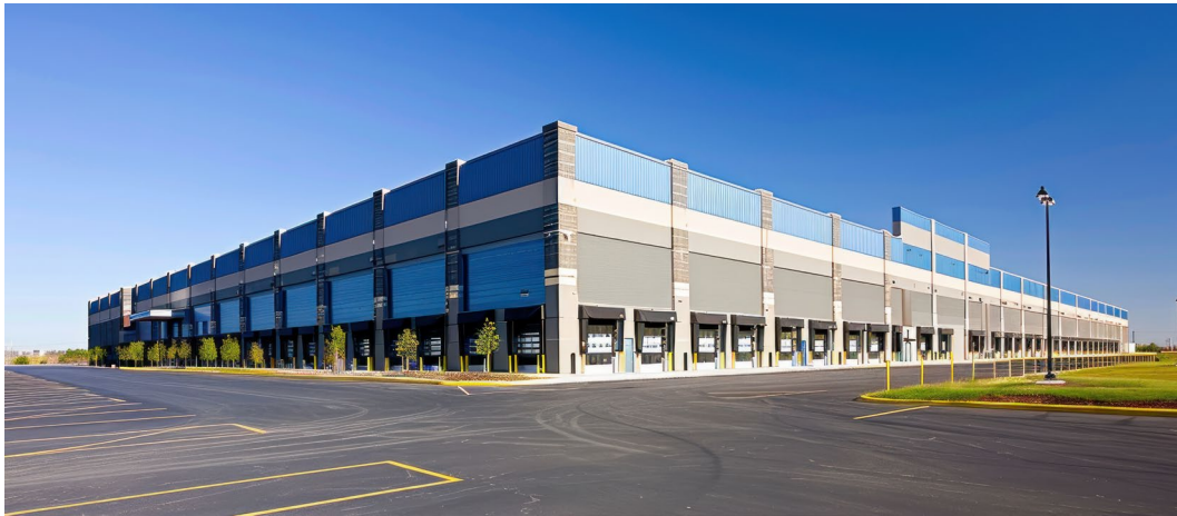
Figure 6.2-2: Illustration of how the façade design requirements such as columns may be applied to industrial buildings.
