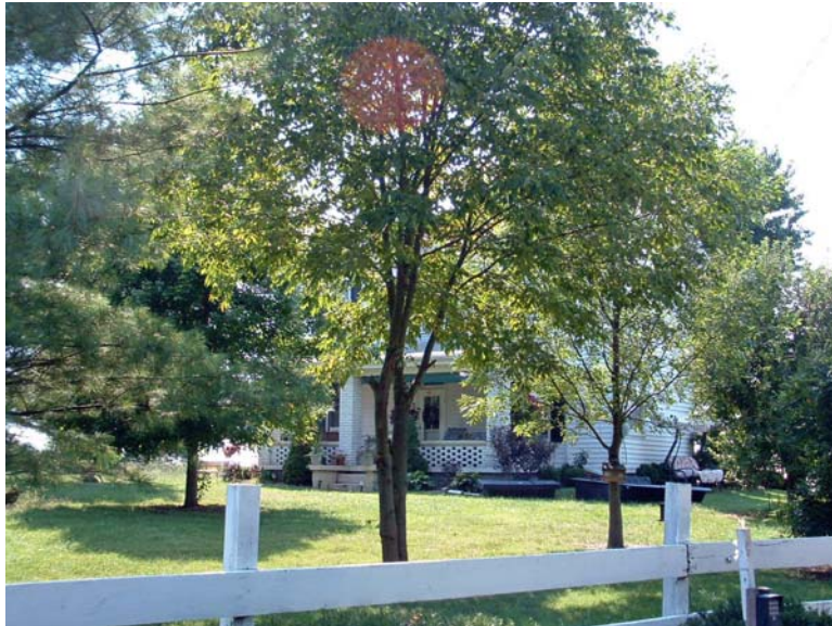
66. 5019 Yankee Road, parcel D2010-020.000-018 Constructed in 1900, Murphy residence/Connie F. Grooms TR home and farm
