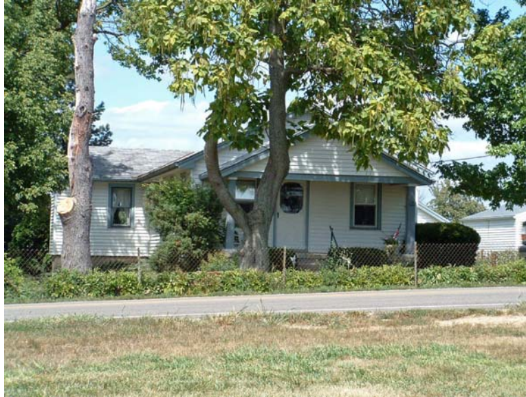
17. 4812 Millikin Road, parcel D2020-031.000-002 Constructed in 1926, Rueben E. and Geneva A. Kadle home
