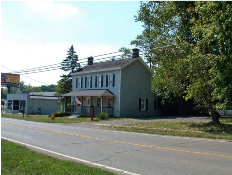
56. 6551 Cincinnati Dayton Road, parcel D2030-050.000-029 Constructed in 1905, Reis residence/Bertal/Crane/Hair/Rush/John Prather house
