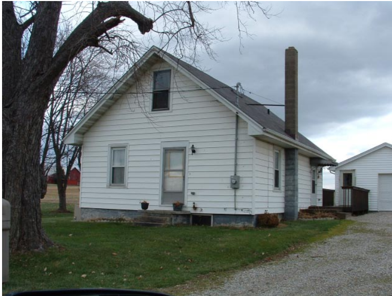
77. 5200 Millikin Road, parcel D2010-003.000-006 Current home of Mark and Sonya Smith, constructed in 1940, tenant home on Munafó's farm
