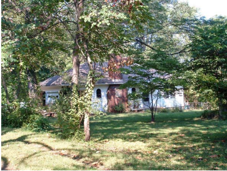
37. 5721 Princeton Glendale Road, parcel D2020-030.000-020 Gilchrist residence/Herman summer residence
