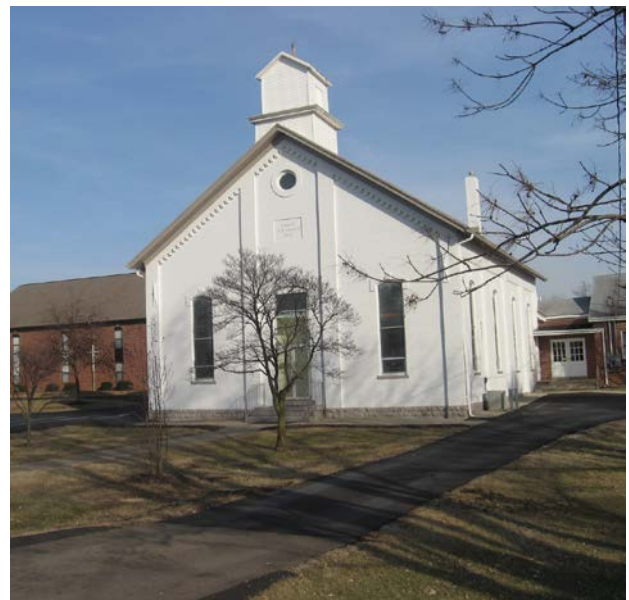
Fig. 3. Bethany United Methodist Church, built 1875 in Bethany
