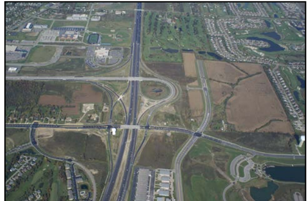
Fig. 20. Aerial photograph of Liberty Way Interchange at the opening in 2009.
